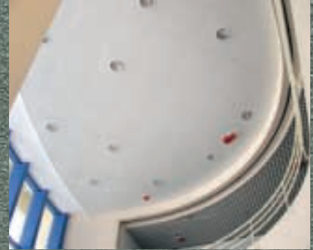
天水圍111區二座興建中之小學天花 Ceiling for construction of 2 primary schools in Area 111, Tin Shui Wai
