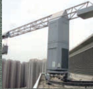
天水圍嘉湖海逸酒店永久吊船 Permanent Gondola at Harbour Plaza Resort City, Tin Shui Wai
