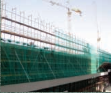
荔枝角九巴車廠平台地盤 KMB Depot Prodium Site at Lai Chi Kok
