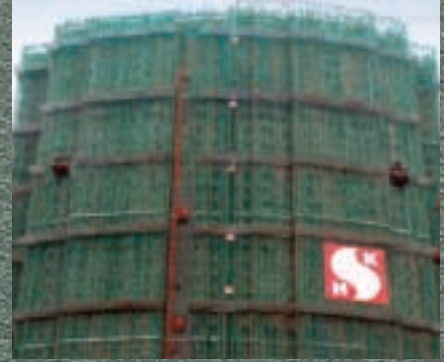
荃灣市373地段(楊屋道)項目 Tsuen Wan Town Lot No.373 (Yeung Uk Road) Project
