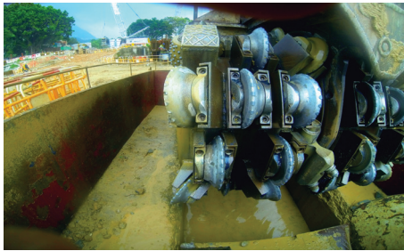
Roller cutters to diaphragm wall
