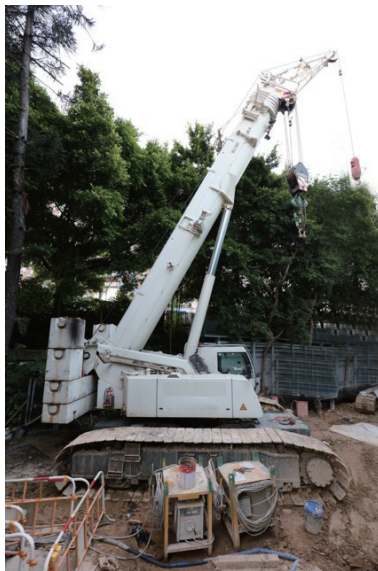
Crawler crane with telescopic boom
