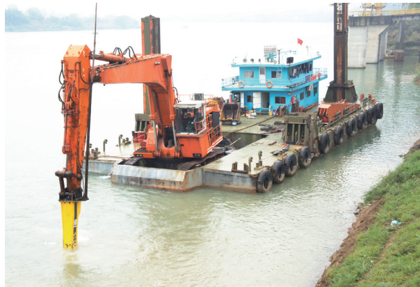
Underwater hydraulic breaker
