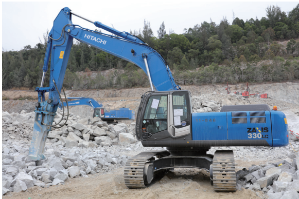
Excavator with hydraulic breaker
