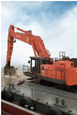
Dredging excavator of 120-tonne class
