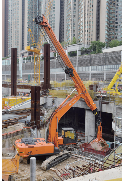
Excavator with 30-metre telescopic arm and clamshell bucket with slide cabin
