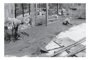
Floor screeding works refer to the application of a well-blended mixture of cement with graded aggregates and water to a floor base in order to form a sturdy sub-floor for the completion of the final floor. If there is pipe-work in the screed, we would ensure that there
