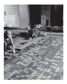
Tile laying works refer to a series of tasks to be performed in a proper sequence in order to lay the tiles on the surface of a wall or floor. Checks are conducted to see whether there is any unintended colour/shade variation within the tiles. We also check whether the adhesive to be used is compatible with the background/base of the wall/floor. Tiles would be
