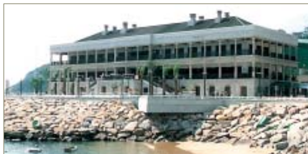
Murray House reconstructed by SOCAM won the "Special Architectural Award-Heritage" at the Hong Kong Institute of Architects Annual Awards 2001
