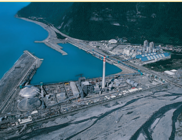
Ho-Ping Power Station, Taiwan
