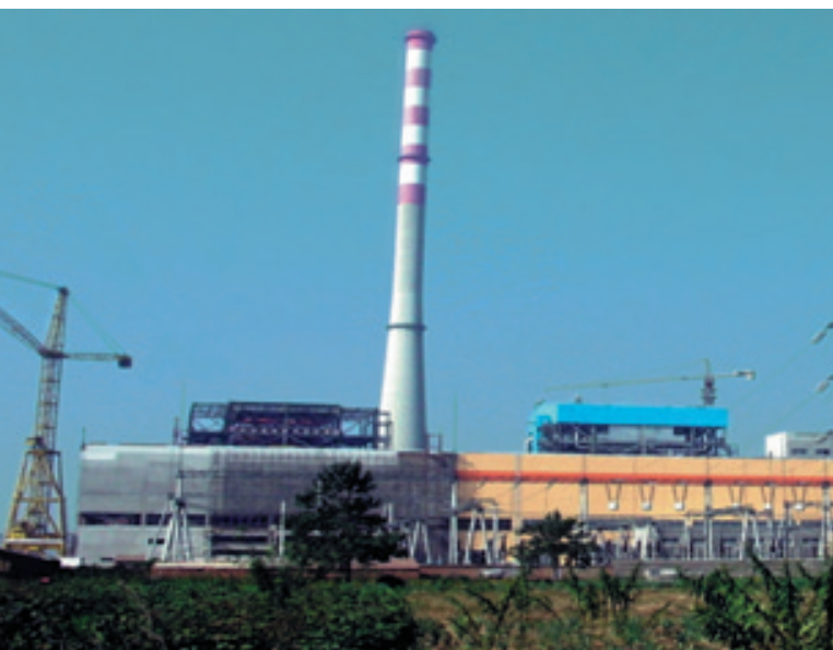
Heze II Power Station, Shandong Province, China
