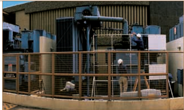
Installing active noise control on a transformer
