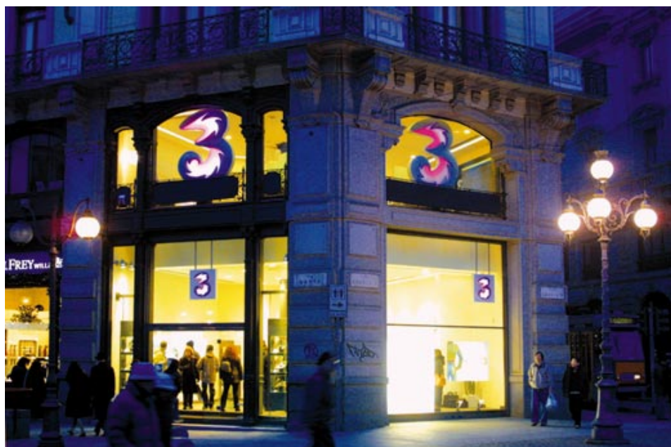
Night view of the two-storey Negozio 3 located in the heart of Milan.
