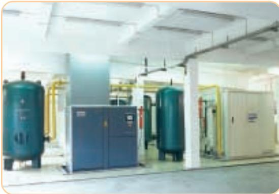
**Nitrogen Generator for Lead Free Soldering**
