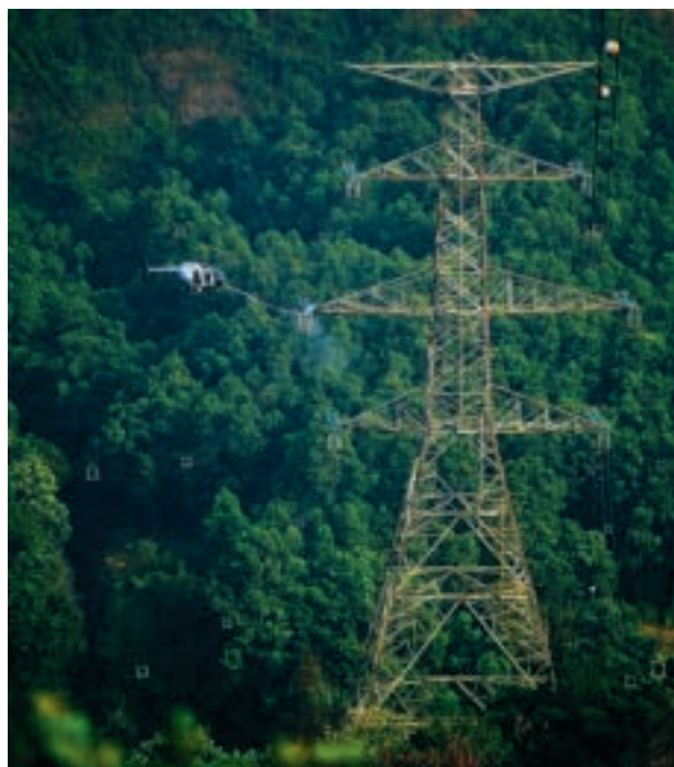
In February 2003, CLP introduced high voltage line cleaning by helicopter – improving speed and efficiency
