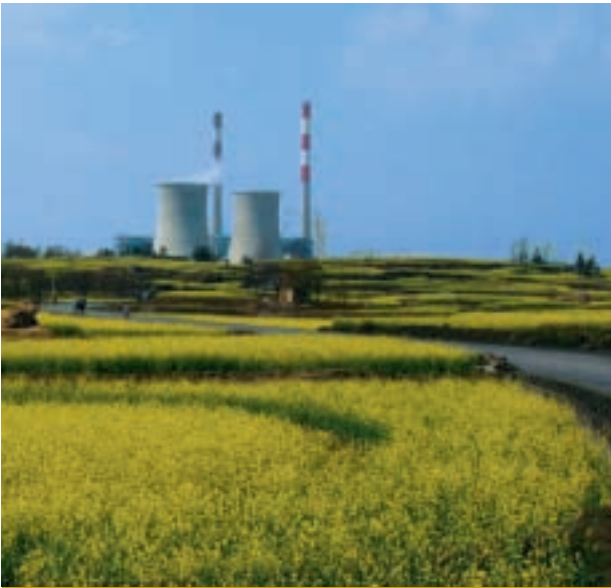
Anshun Power Station – Unit 1 started trial operation in March 2003
