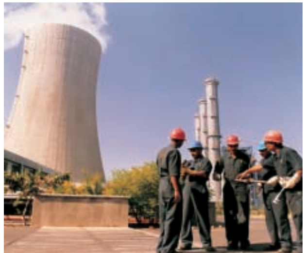
GPEC – now 100% owned by CLP
