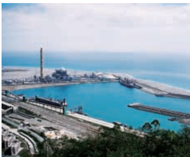
A 250-metre chimney towers over the newly operational Ho-Ping Power Station on Taiwan's east coast
