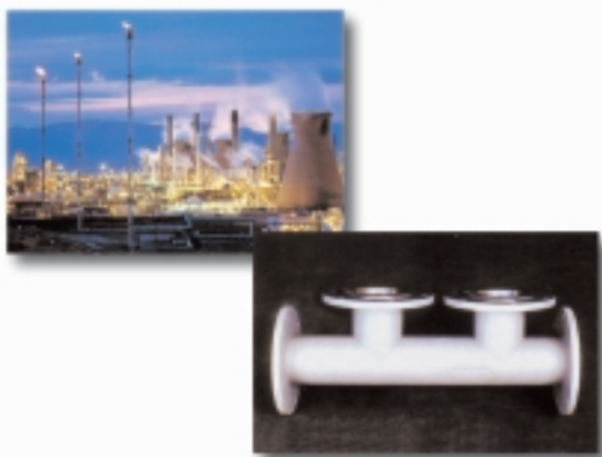
Petrochemical plants and energy saving device
