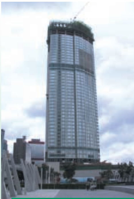
PABX System Solution for Four Seasons Hotel at Hong Kong Station Development
