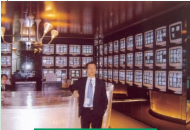
Mr. PK Fung, Managing Director of the Group, in the control room of Digital Surveillance and Security Systems at Two International Finance Center
