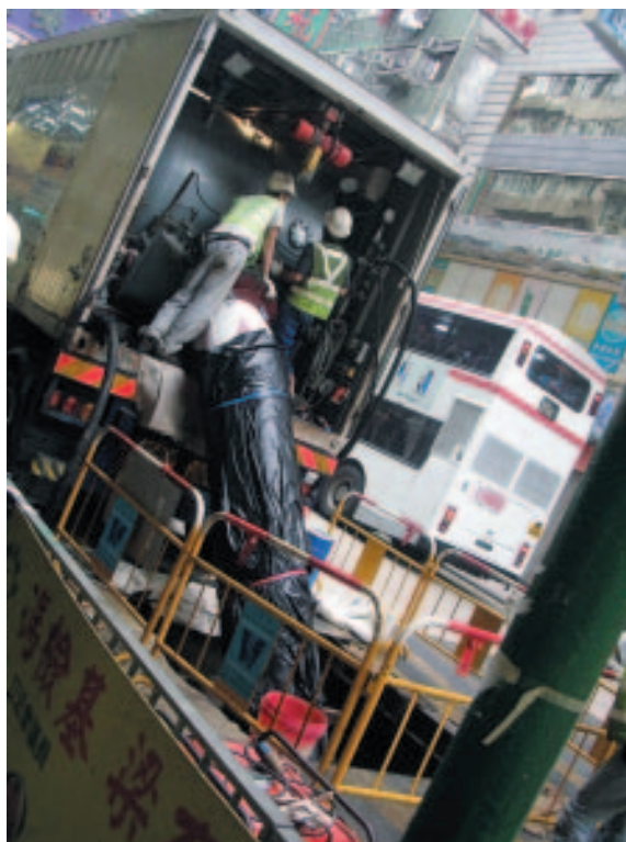
Rehabilitation of a DN600 Fresh Water Main at Castle Peak
