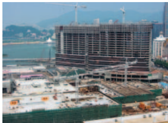
Mechanical installation at Wynn Resorts in Macau
