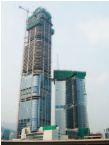
Installation of lifts and escalators and curtain walls at Nina Tower
