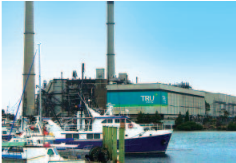
1,280MW gas-fired power station at Torrens Island, South Australia
