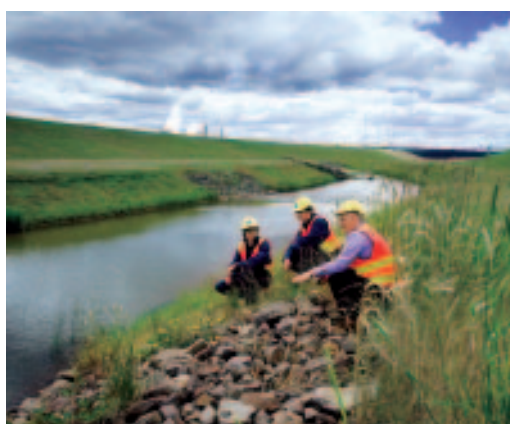
Morwell River Diversion Project – before, during and after (from left to right)
