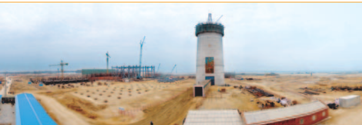
Fangchenggang project – well on track
