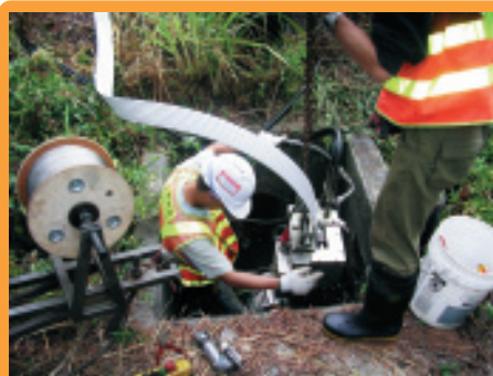
Ribloc installation at Hung Shui Kiu
