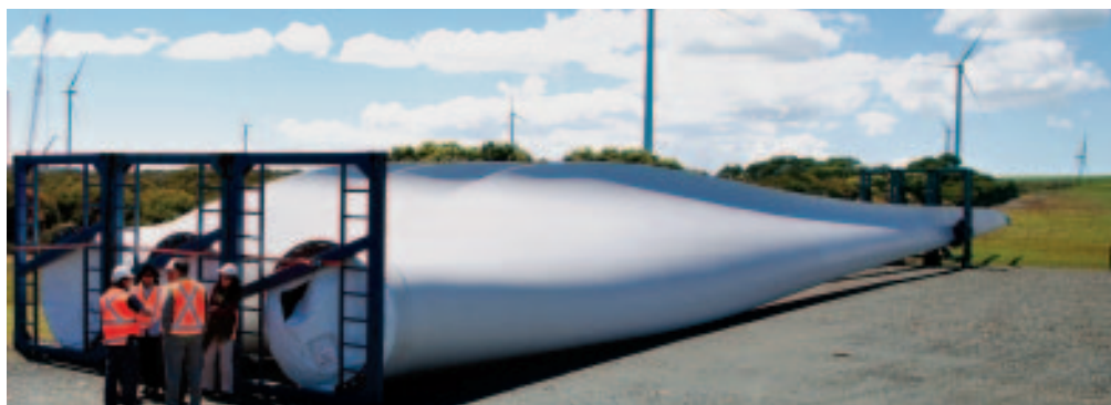
→ Wind turbine blades ready for mounting at Woolnorth Bluff Point, Tasmania
