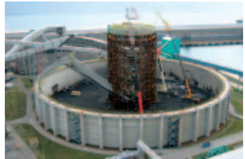
← Rebuilding a damaged coal dome at Ho-Ping Power Station, Taiwan →
