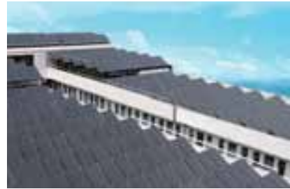
Solar Energy Panels
