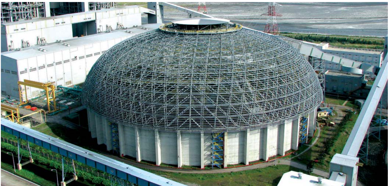
○—○ Ho-Ping: Coal Dome C under construction
