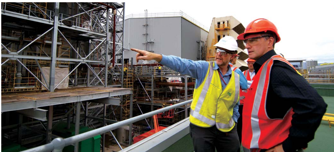
○—○ Inspecting construction progress of Tallawarra Power Station
