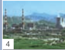
4 Shang'an Power Plant (1,300 MW)
