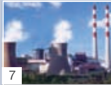
7 Yushe Power Plant (800 MW)
