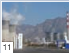
11 Qinbei Power Plant (2,400 MW)
