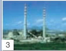
3 Dalian Power Plant (1,400 MW)
