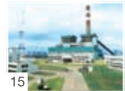
15 Shanghai Shidongkou Second Power Plant (1,200 MW)
