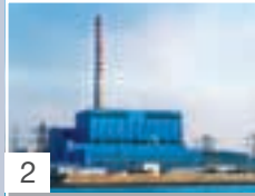
2 Yingkou Power Plant (1,840 MW)
