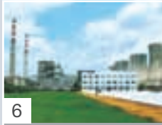
6 Dezhou Power Plant (2,650 MW)
