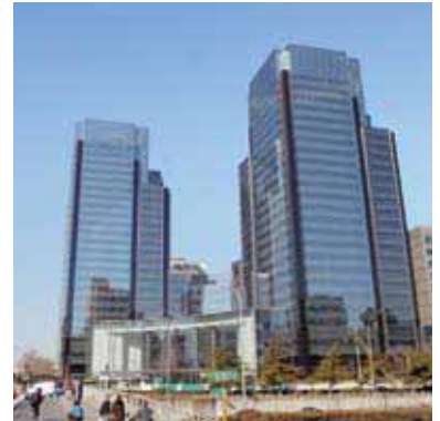
Huapu Centre (Phase I)
