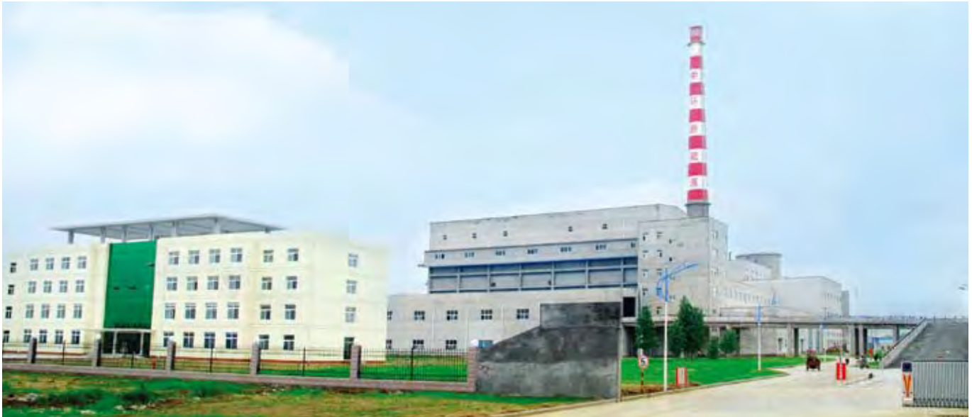
Linyi Power Station Shandong China
