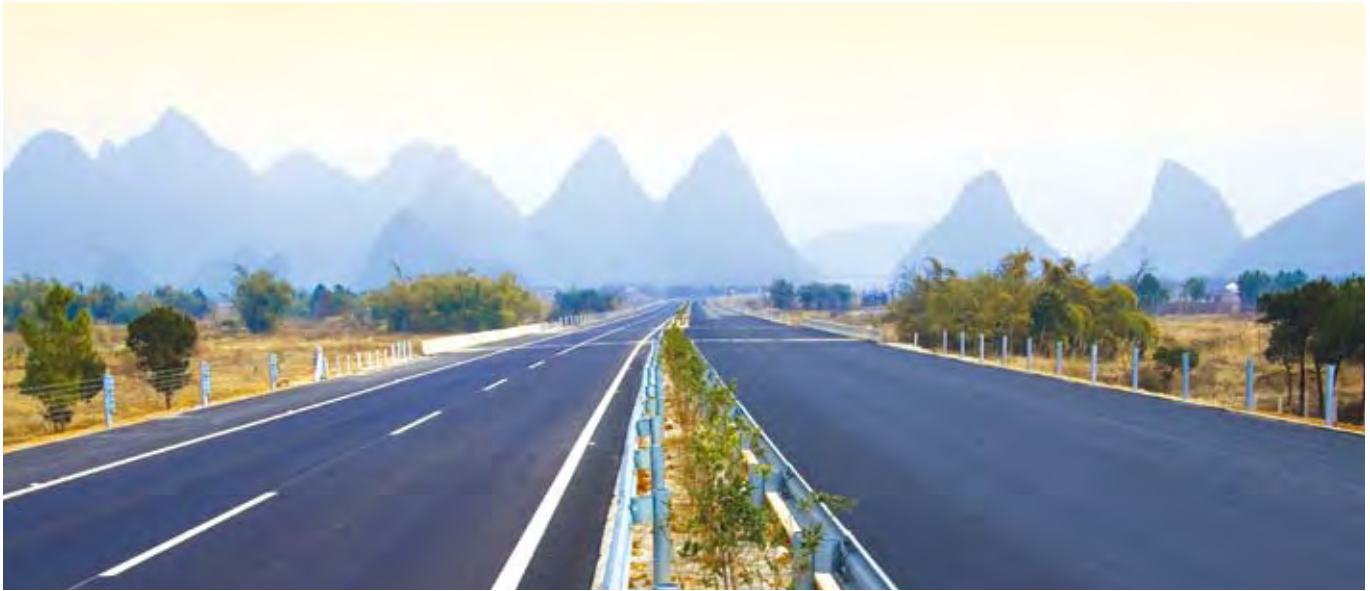
Toll Road of Guilin, Guangxi
