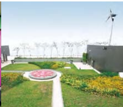
The Marsh Road Station Building adopts a green building concept.
