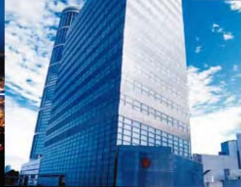
Tamar is one of several major transmission projects completed in the past year.
