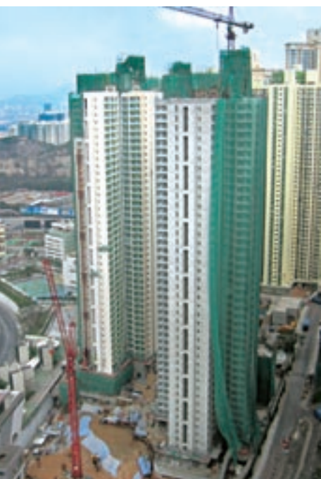
Eastern Harbour Crossing Site Phase 4
