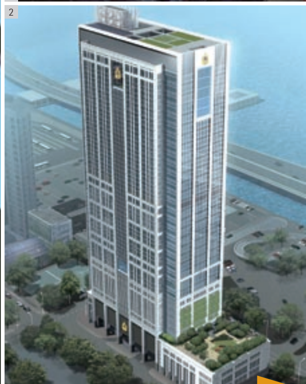
1. ICAC Headquarters Building 2. New Headquarters of the Hong Kong Customs and Excise Department
