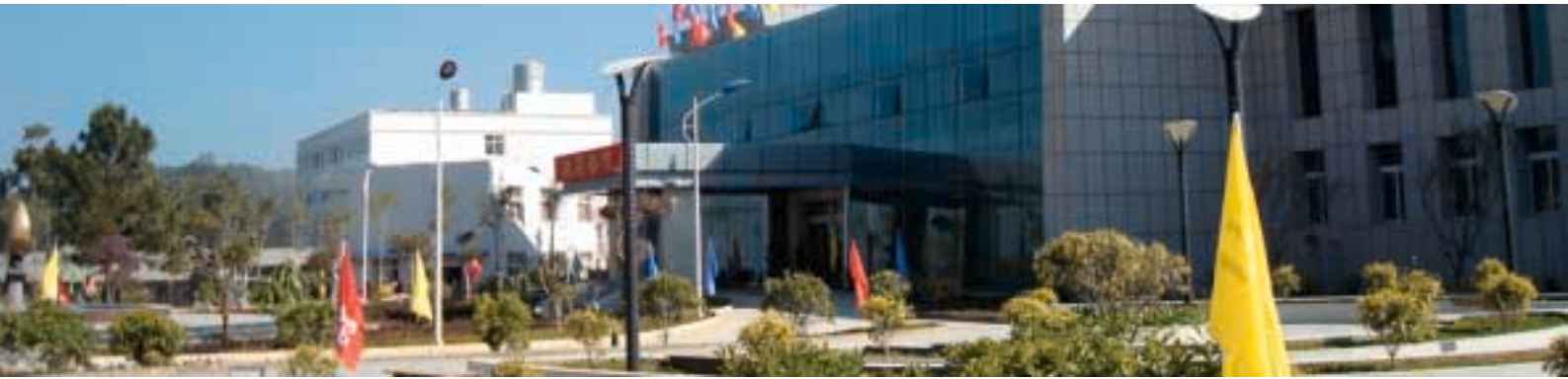
Dapingzhang Mine Office & Accommodation
