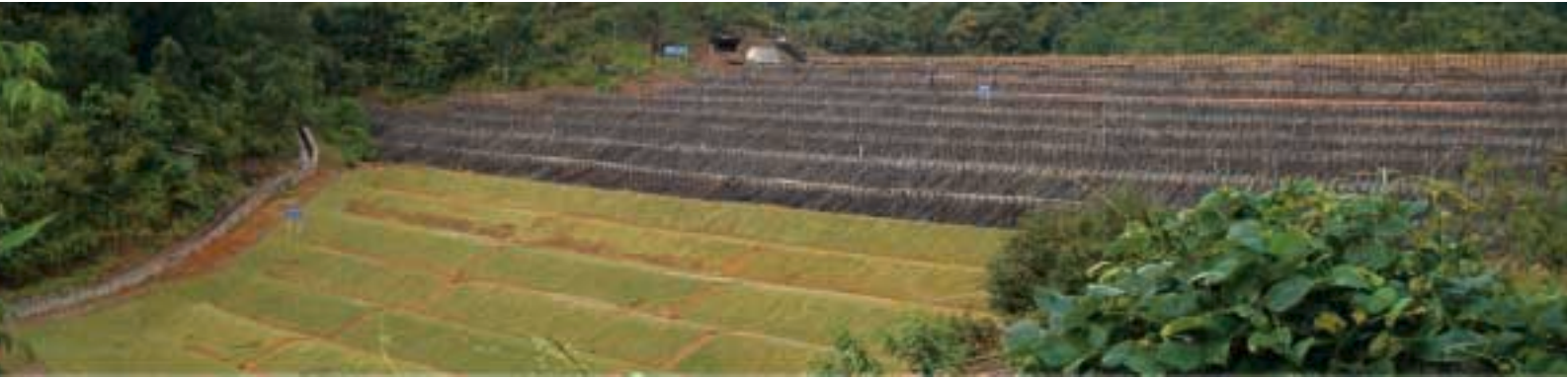
Revegetation of Tailings Dam Wall at Dapingzhang
