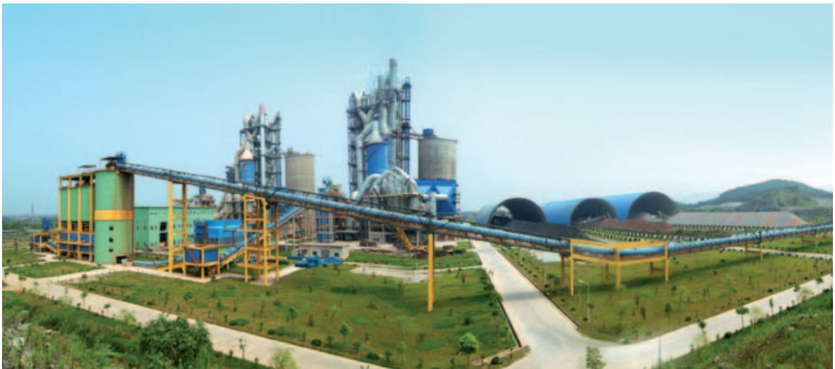
Clinker production base of Zhejiang Cement with a daily capacity of 10,000 tonnes
