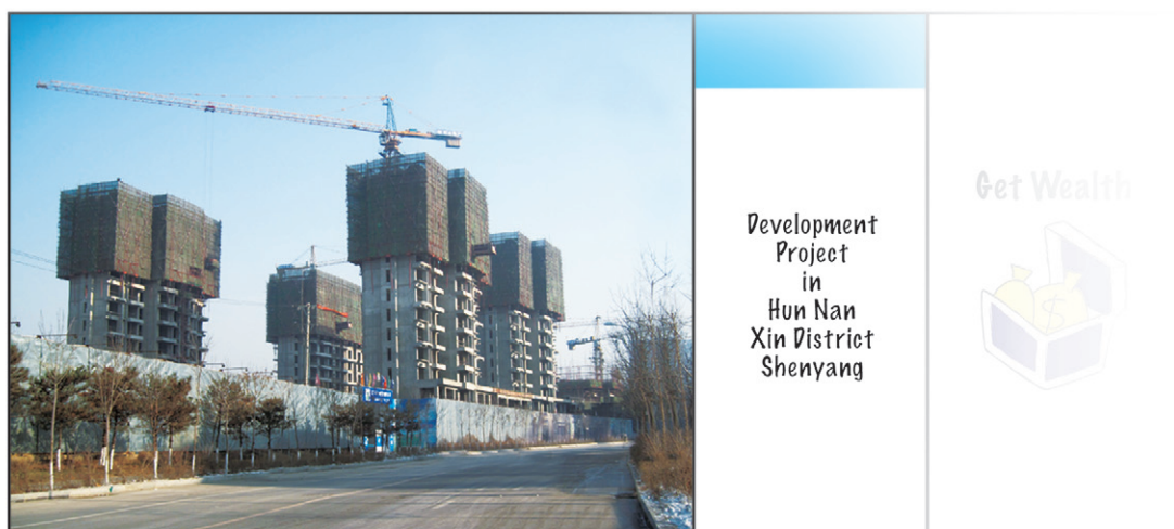
Construction works in progress
