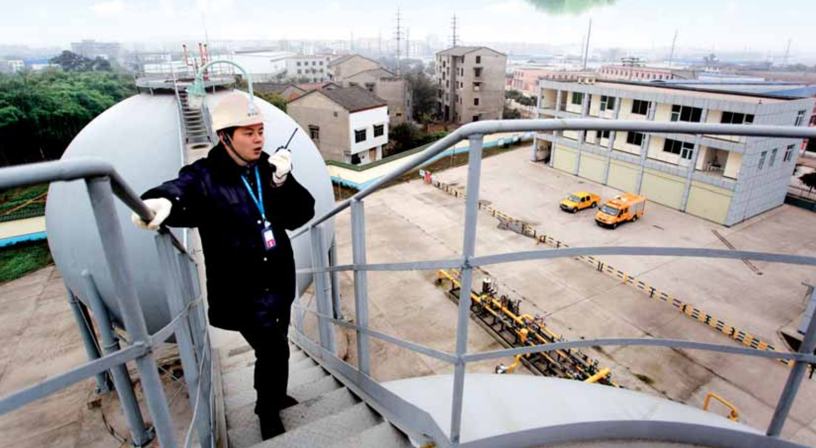
Technicians carry out regular safety inspections against gas leakage for pipelines and facilities.
