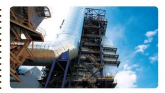
An FGD plant and a Low NOx Burner system have been installed for the coal-fired generating unit L5.
