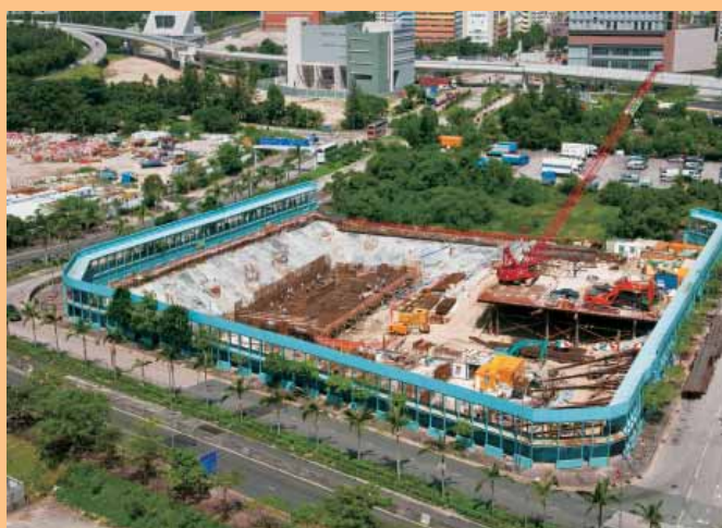
Works at West Kowloon Reclamation Area 西九龍填海區之工程
