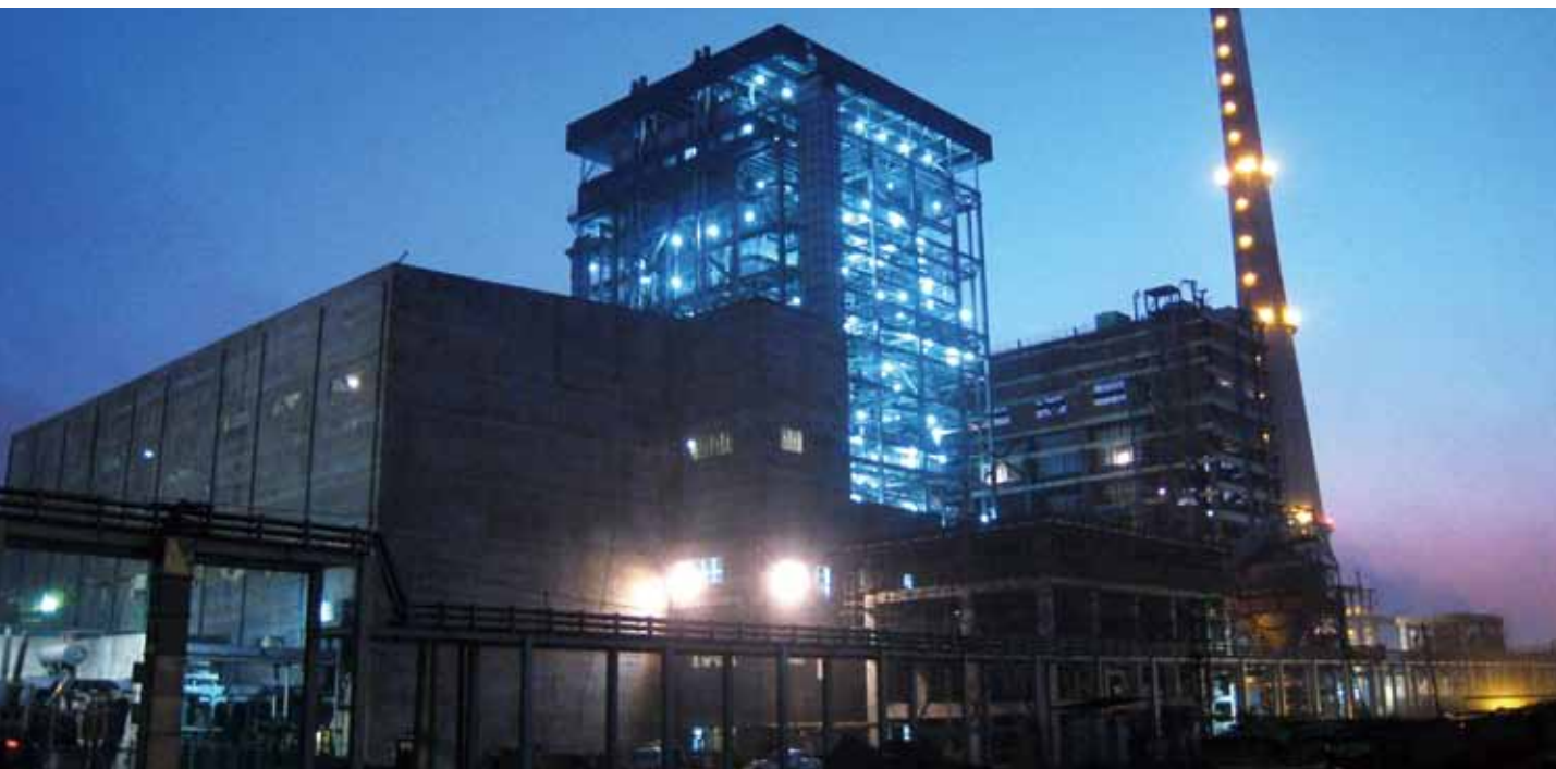
India Dugarpur power plant project
