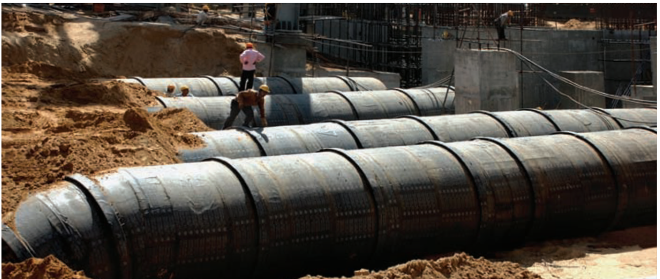
Construction workers placing cooling water pipelines at the Mahatma Gandhi Thermal Power Plant, Jhajjar
