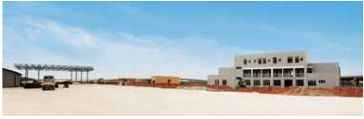
Exit to Fortune Wealth Memorial Park from highway linking Guangzhou to Hezhou, with toll station under construction
