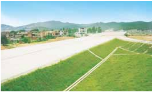
Highway linking Guangzhou and Hezhou, near completion stage
