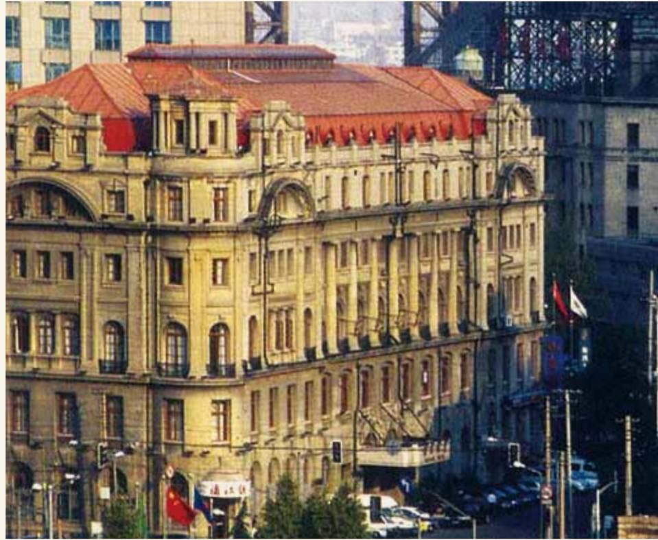
Above : The Astor House Hotel today. The building still retains many elements introduced in the 1920s and continues to provide accommodation for visitors to Shanghai.
