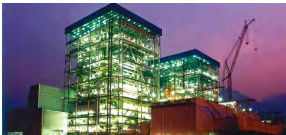
The first 600MW super-critical boiler of Qinbei Power Plant in the PRC
