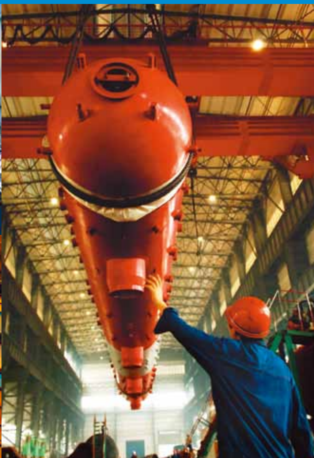
Hoisting and installation of power station boiler
