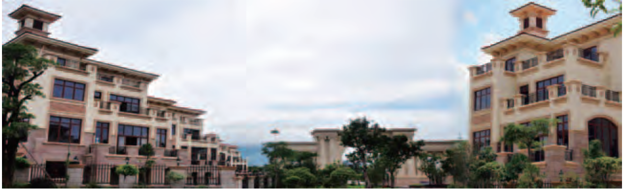
Completed Villas in CSC Heyuan 河源華南城已建成之別墅
