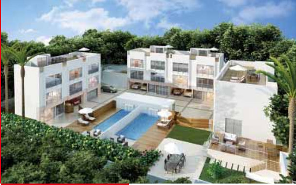
684 Clear Water Bay Road, Sai Kung, Hong Kong
