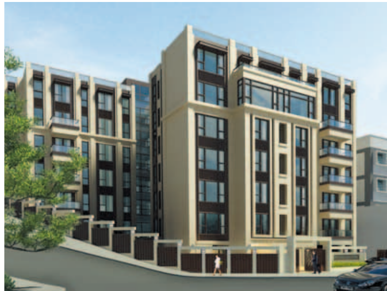
▲ Tai Hang Road Project
