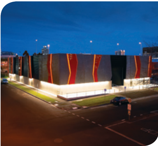
Citipower's award-winning Southbank Zone Substation features an innovative exterior design and utilisation of modern GIS technology.
