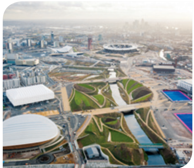
UKPN stands ready to power the 2012 London Olympic and Paralympic Games.
