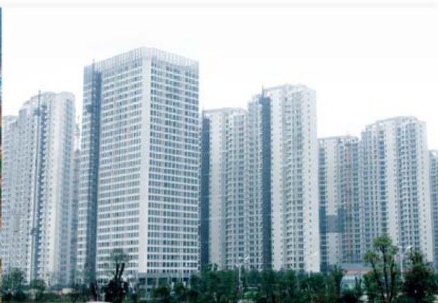
▲ CSC Nanchang residential facilities 南昌華南城住宅設施
