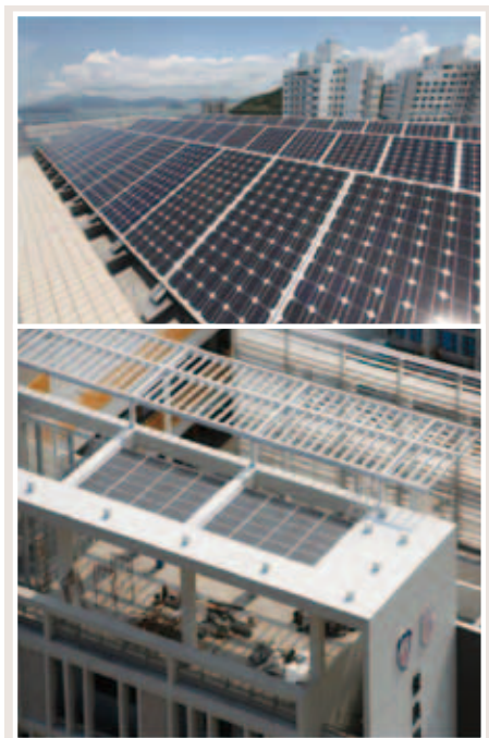
PV Panels at Li Shu Fan Building, HKU and So Kwun Wat Primary School 香港大學李樹芬樓及掃管笏小學之太陽能面板
