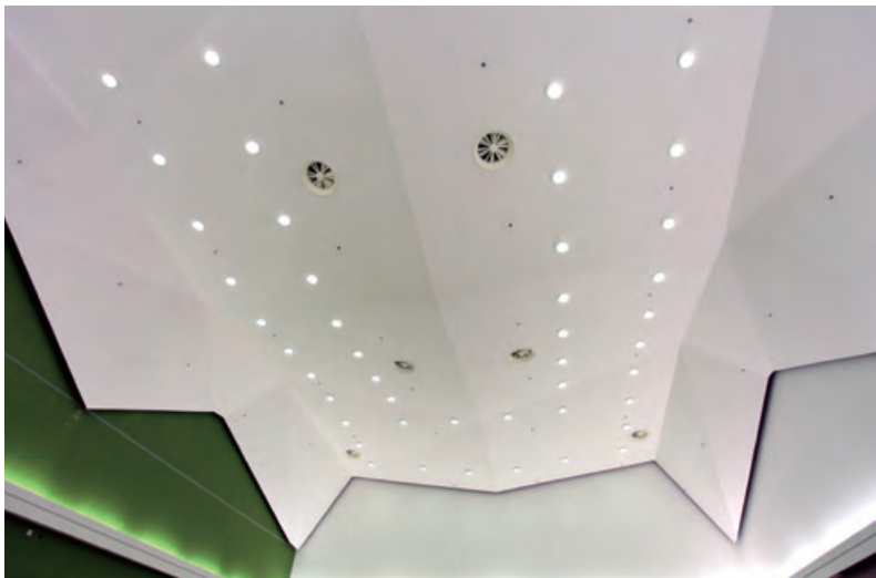
Lam Tin North Municipal Services Building – False ceiling 藍田北市政大樓—假天花系統
