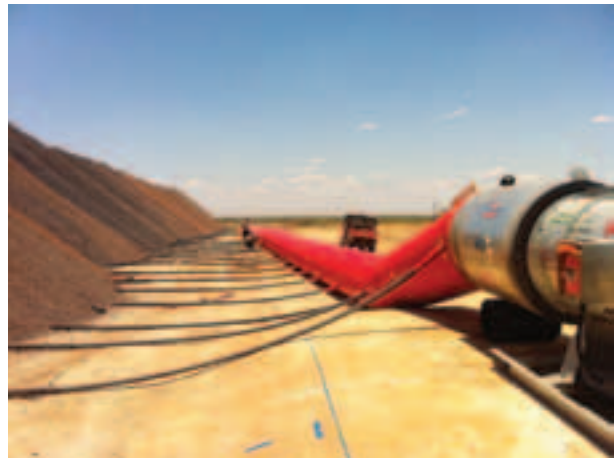
Figure 6: leach heap forced-aeration equipment
