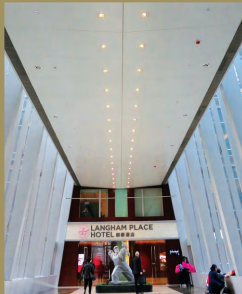
RETROFITTING OF LED LIGHT FITTINGS
