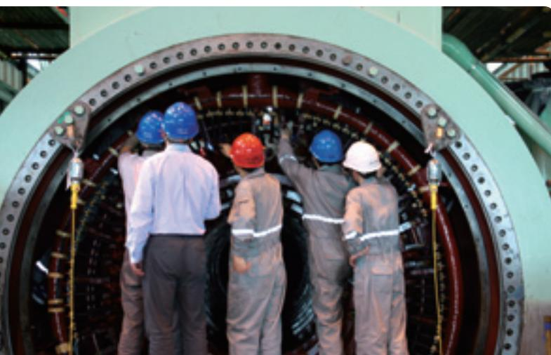
▲ Jinwan Power Plant engineers overhaul Unit 4 generator to enhance overall reliability and efficiency.
