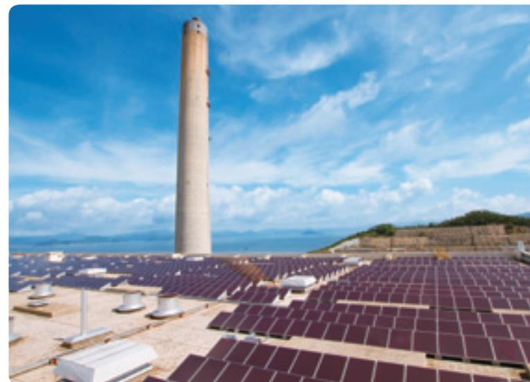
▲ With over 8,600 thin-film photovoltaic panels, the solar power system at Lamma Power Station is the biggest in Hong Kong.
