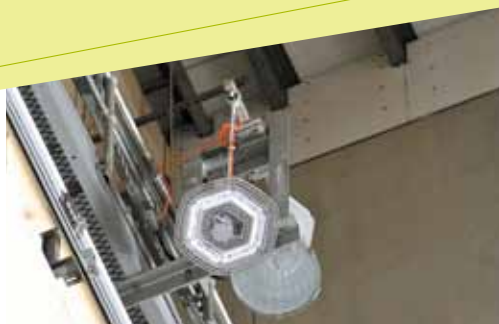
Old metal halide lamp (right), new LED light (left)
