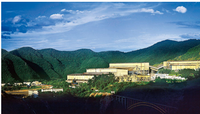
Copper mine processing plant in Jiangxi Dexin
