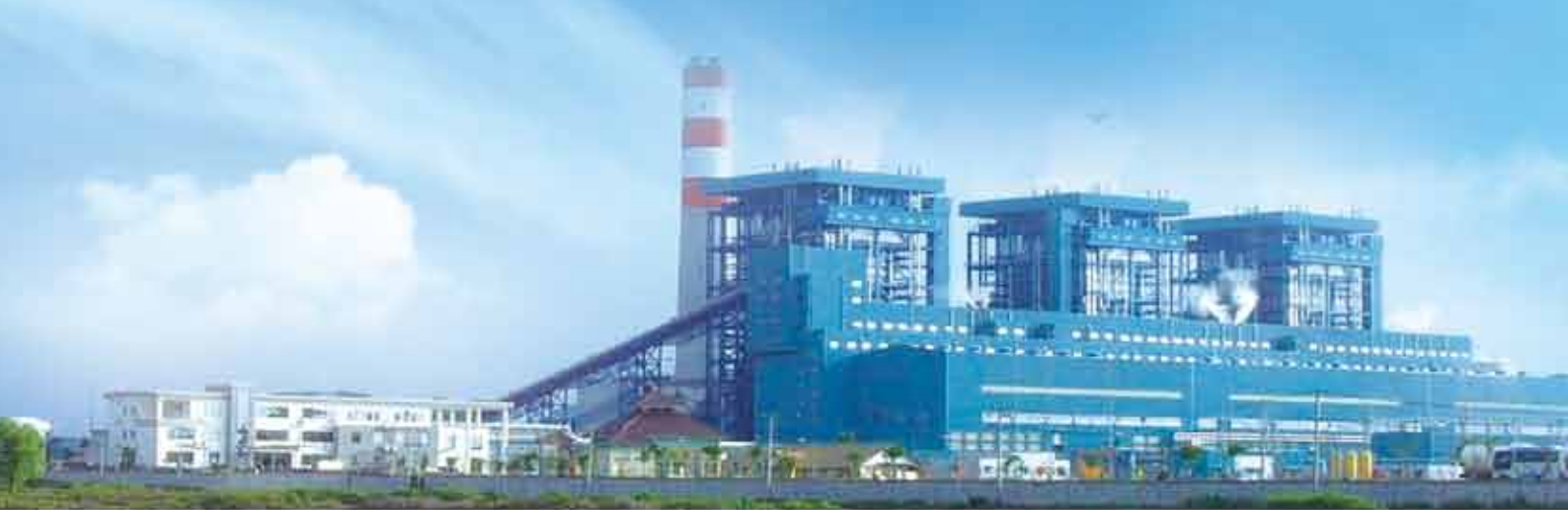
Longwan Power Plant in Indonesia, constructed by the Company
